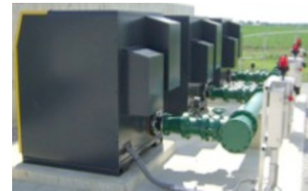
AS aeration tank pumps
